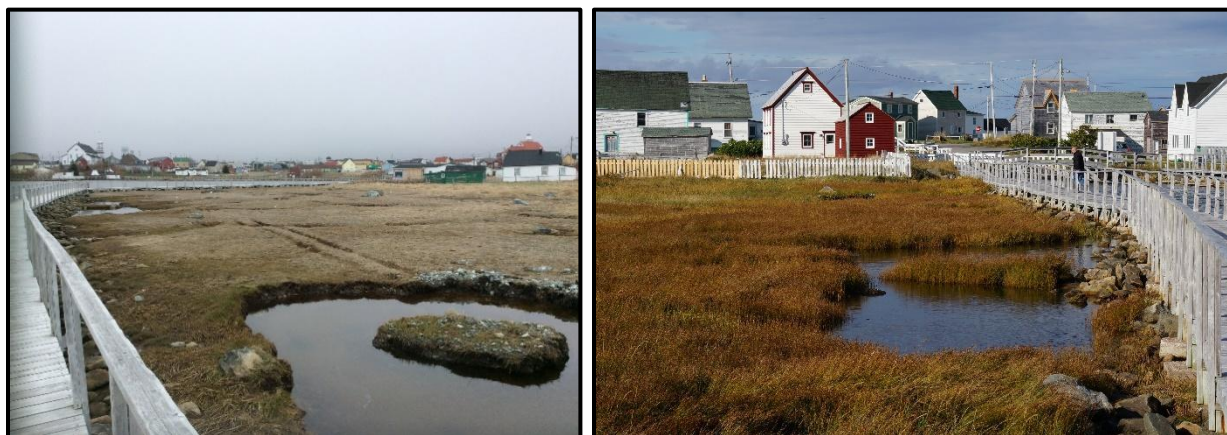
Lefthand photo: Construction in progress to dig out a former wetland and recreate islands; righthand photo: At the conclusion of the project - one of the completed islands showing new growth. Staff photos
