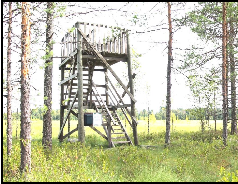
Figure 7. A wooden bird viewing tower Photo from Creative Commons
