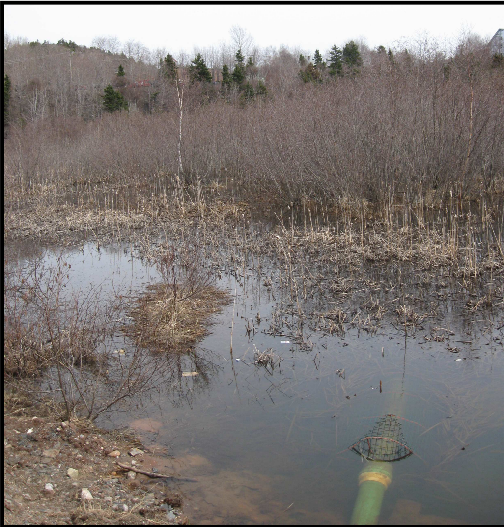
Figure 5 – Water Control Structure installed by Ducks Unlimited Canada at the Glynmill Inn Marsh, Corner Brook. Photo by Charmaine Barney
