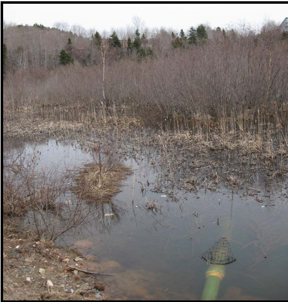
Figure 8 - Water Control Structure installed by Ducks Unlimited Canada at the Glynmill Inn Marsh, Corner Brook. Photo by: Charmaine Barney
