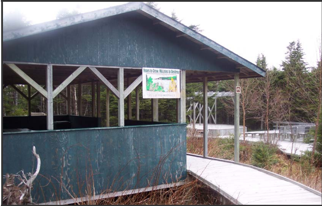
Figure 1 – Ecomuseum Shelter and Amphitheatre in Winterland Photo by EHJV Staff
