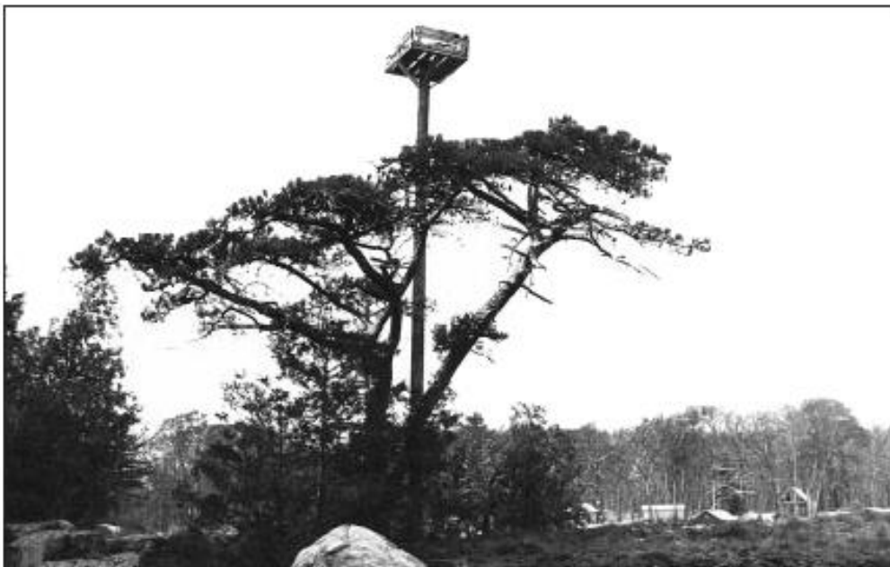
The single-poled platform is designed for use on land. It can be erected in deep soil or on rock.
