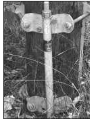
The pole is anchored with a mounting set.
