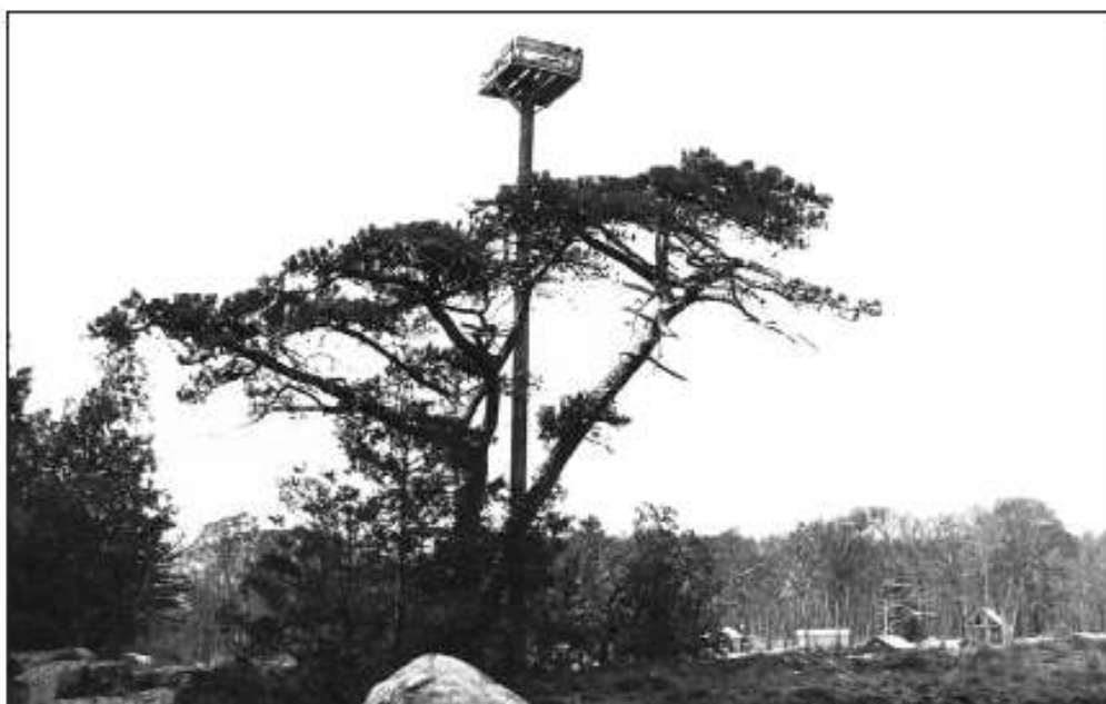
The single-poled platform is designed for use on land. It can be erected in deep soil or on a rock.
