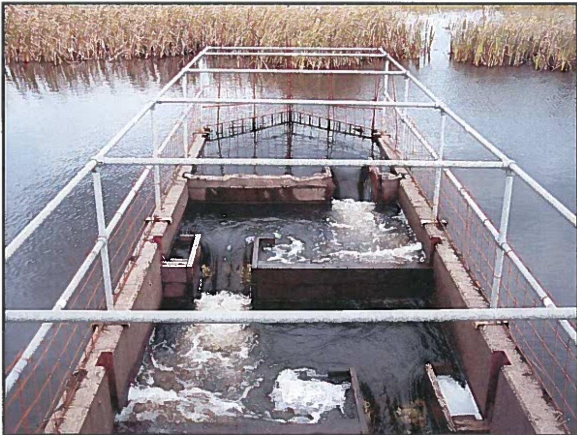
Image 10: Fish Baffles in Grand Falls – Windsor, NL. Photo by: NL Wildlife Division
