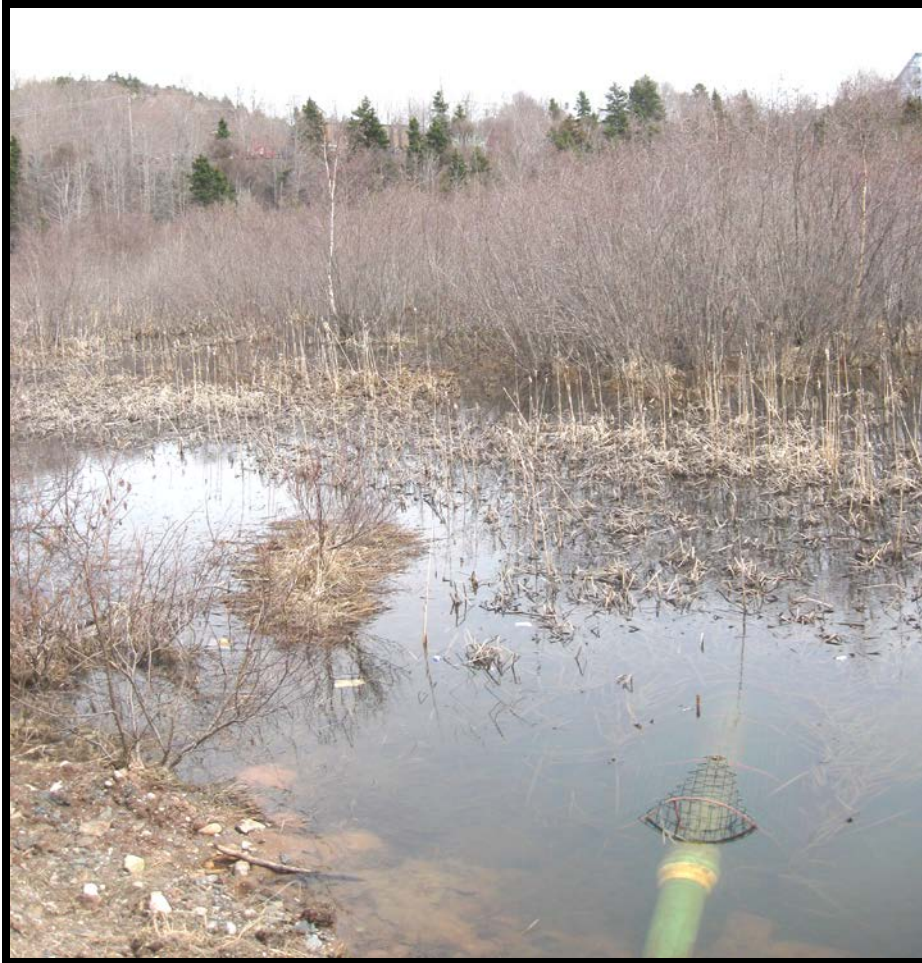
Figure 22 - Water Control Structure installed by Ducks Unlimited Canada at the Glynmill Inn Marsh, Corner Brook. Photo by: Charmaine Barney
